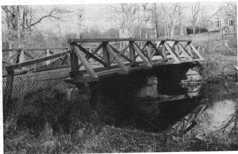
Dugway Bridge: Dugway Bridge Road. (#31)
