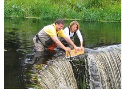
Engineers Jim MacBroom and Jeanine Bonin conduct a dam inspection of Horseshoe Falls as part of the Shannock Fish Passage Feasibility study.
