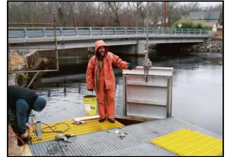
Workers for RI Department of Environmental Management install a new gate and platform at the Potter Hill Fish Ladder on the Pawcatuck River.
