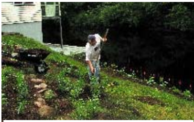
Restoring the bank of the Wood River at the WPWA campus.
